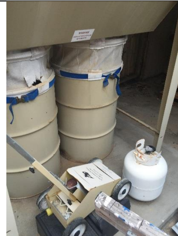
Dust collector on east side of building.
