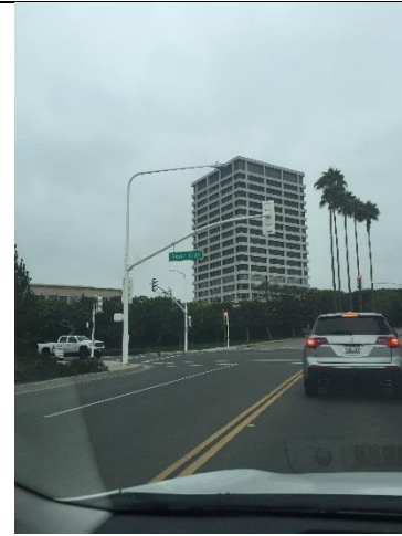
Eastern adjacent property.
